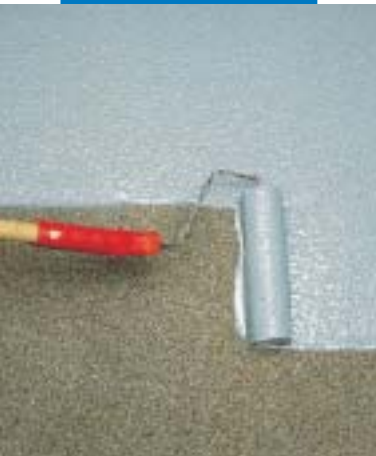
Applying Mapecoat I 24 with roller
