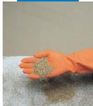
Spreading dry sand on fresh Mapecoat I 24
