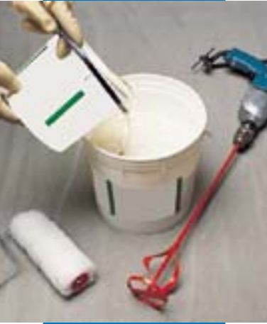
Mixing part B with part A
