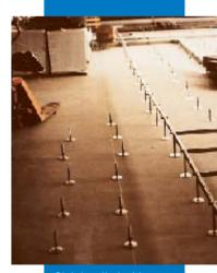
Slab levelled with Ultraplan ready for fixing a floating floor
