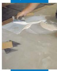
An example of an installation of inlayed PVC on a surface levelled with Ultraplan - CD2 - Milan - Italy
