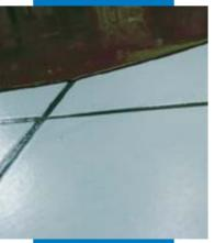
Detail of the application of Ultraplan on an existing ceramic tile filoor after the application of Mapeprim SP
