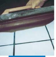
Application of Ultraplan with a metal trowel on an existing ceramic tile floor after the application of Mapeprim SP
